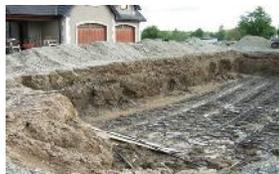
Buried piping for external heat exchange
