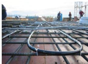
Heating/cooling pipes to be embedded into concrete floor with the rebar
