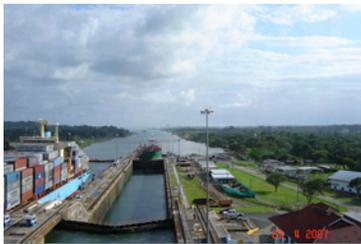
some of the water that is flushed out each time a ship passes through a lock. This water will then be used to partially refill the lock for the next ship.
