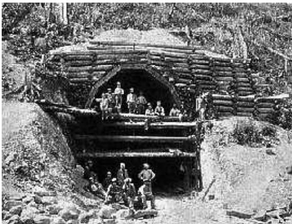
The mine portal is the original opening to the Balmer coal mine in Natel, BC about 1904. The shape is to provide for pressurized ventilation with fresh air from surface. The practice is to avoid moving coal mine exhaust over mechanical fans with risk of sparks in an explosive atmosphere. For further reading on this fascinating storey, please refer to [www.wcgce.org](http://www.wcgce.org) under Past Events/AGM2014
